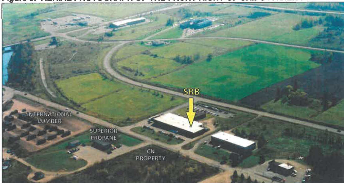
Figure 3: AERIAL PHOTOGRAPH OF THE FRONT RIGHT OF SRB'S FACILITY
